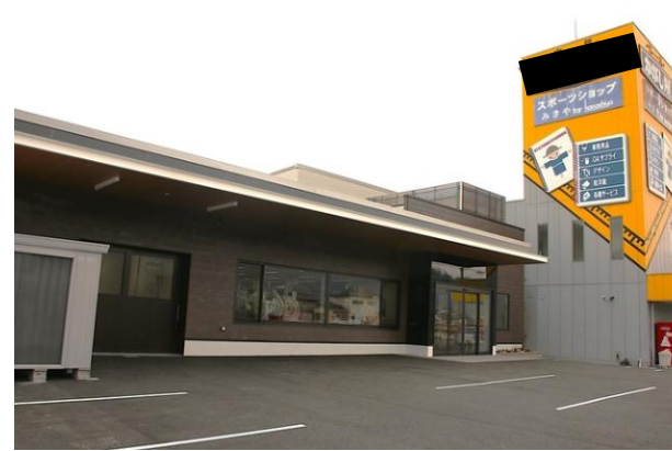
The new company building will be raised by 80 cm
